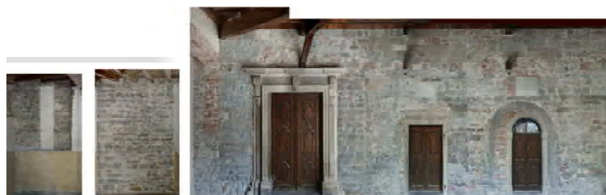
Façade of the Church of S.Giovanni after the plaster removal
